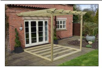
Add the remaining rafters, using the markings on the runner and wall plate to align them before securing in place with 2 x 120mm coach screws as per the outer rafters.
