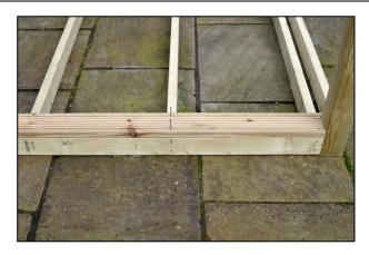
Work your way down the edge section, keeping it flush with the frame and using the joists as a guide, affix in place with 2 x shorter screws at every joist. Repeat Steps 20 -22 for the other decking edge section.
