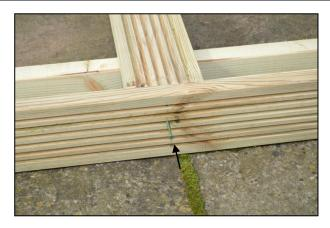
Using the decking section that you placed centrally earlier as a height guide, fix the centre of the front cladding in place, flush with the top surface of the decking using a shorter green screw.
