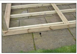
Add intermediate screws through the front cladding into the frame.
