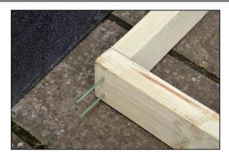
Butt the end of the joist closest to the wall up to the end of the side frame, make sure everything is flush and aligned and then screw through the pre-drilled holes in the side frame into the joist end using 2 x longer green screws. Repeat for the other side.
