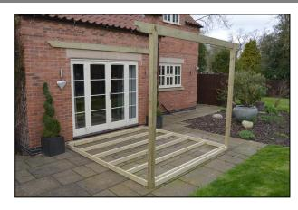
With the help of an assistant, slot the remaining runner into the top of the posts, using the markings on the runner to correctly align it centrally across the structure.
