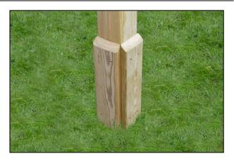
Attach the optional Pedestal panels to the bottom of each post as shown. Line up each panel on the post so that it is flush with the bottom face and secure each one into place with 4 x woodscrews.
