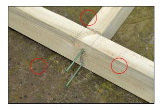
Line up the end of each joist end with the markings on the side frames, making sure the top faces are also flush, before screwing into place with 2 x longer green screws.
