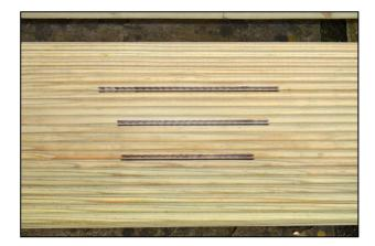
Identify the side cladding panels with the 3 parallel lines as shown here.
