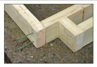
Attach the base frame sides to the base front assembly using 2 x longer green screws in the predrilled holes, making sure that the ends are flush and everything is square. Repeat for the other side frame.
