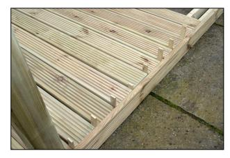
Now lay the decking sections onto the frame, butting the edges of the decking up against the inner face of the front cladding section. If the spacing is irregular, adjust as necessary by eye so that the sections are evenly spaced.
