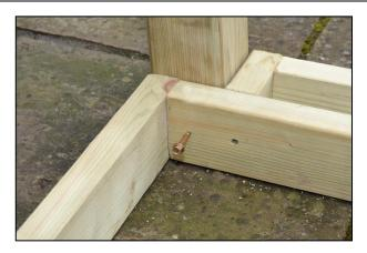
...before securing it into place with a 70mm coach screw through the pre-drilled hole in the frame front assembly. Attach the second post in the same manner.
