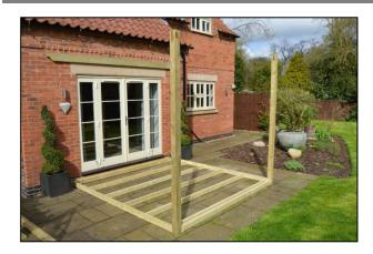
Get an assistant to hold a post upright in the pocket at the front corner of the base frame. Make sure that the notch in the top of the post is correctly oriented so that it is parallel to the wall plate...
