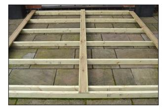
Take one of the decking sections and place it centrally across the joists as shown.
