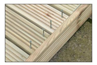
Fix the decking sections into place, using the frame joists as a guide for the screw spacing, with two screws at the edges and at each joist intersection. TIP: If you encounter a decking section that is bowed, simply bend it whilst screwing it into the frame to remedy this.
