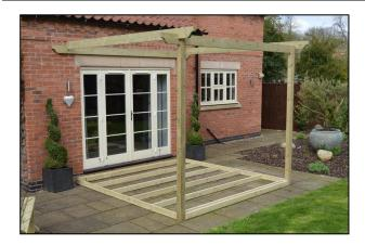
Now sit the outer rafters in place so that the inner face is butted again the post at the front and the rear is resting on the wall plate, aligned with the corresponding markings.
