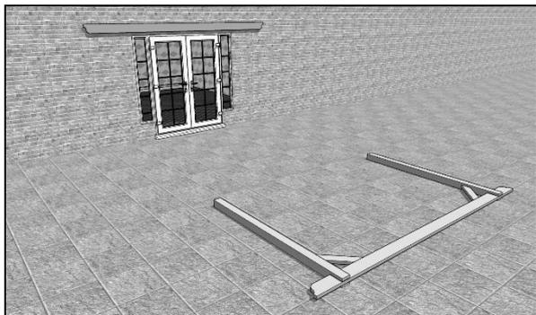
Get your assistants to manoeuvre the previously assembled "goalpost" assembly into place so that it is approximately in place, parallel to and about the length of a rafter away from the wall plate...
