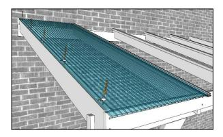
Position one of the drilled polycarbonate panels so that it sits on the glazing bar, aluminium tape at the wall, UV coated side up and the drilled edge flush with the outer rafter. Ensure the inner edge is parallel with glazing bar and adjust the "goalpost" laterally if necessary before fixing the panel in place with 60mm roofing screws and then closing the cover caps.
