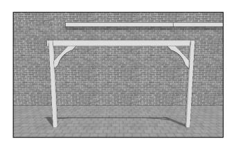
Using your assistants, manoeuvre the previously assembled "goalpost" with 2 posts into place. Position it parallel to the wall with the runner overhang adjacent to the outer end of your wall plates. Consult the Panel length table (page 3) to correctly distance the posts from the wall.
