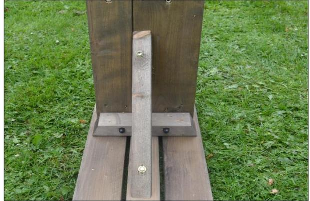
Now attach it to the seat panel and seat end frame using 60mm coach screws.
