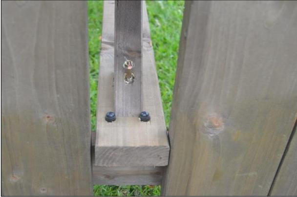
Continue to hold the table leg brace firmly in place and attach it to both the parasol brace and table top using 60mm coach screws. Repeat the process for the other angle brace.
