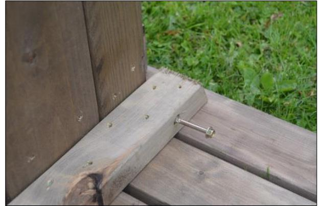
Using one of the supplied 70mm coach screws and the pre drilled holes, secure the table leg frame to the fixing batten on the table top...
