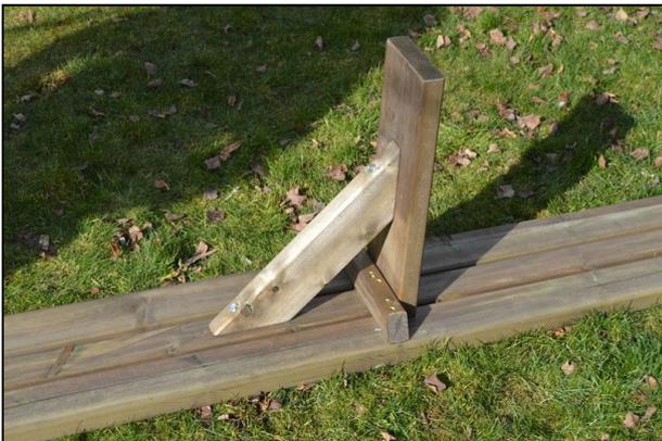
...before fixing into place with a 60mm coach through the brace into both the support and the underside of the seat panel.
