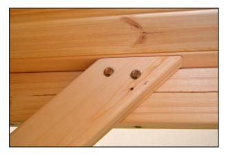
...and the other end is snug against the underside of the bench top. Secure the top of the brace using 2 x 60mm coach screws...
