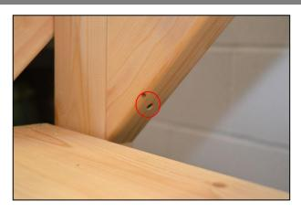
...and the lower end using a 75mm screw as shown here.
