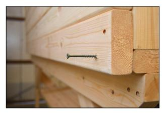
...and secure into place using 4 x 75mm screws. (45mm screws for MDF version)
