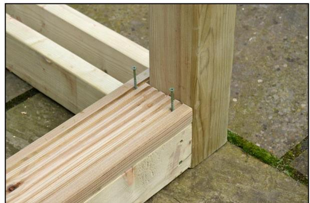
Place the correct Decking edge section in place so that it locates around the post as shown with the decking running front to back and the outside edge flush with the frame edge before securing in place with 2 x longer screws.
