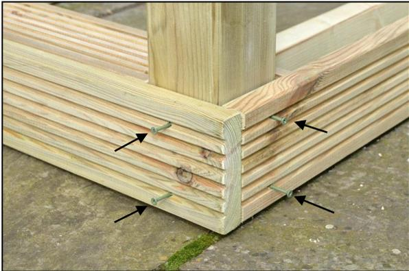
Place the side cladding and front cladding in place and ensure they are flush with both the upper surface of the decking edge section fitted previously and with each other at the outer corner, before securing with shorter green screws as shown above.
