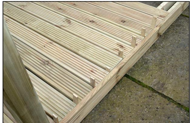
Now lay the decking sections onto the frame, butting the edges of the decking up against the inner face of the front cladding section. If the spacing is irregular, adjust as necessary by eye so that the sections are evenly spaced.
