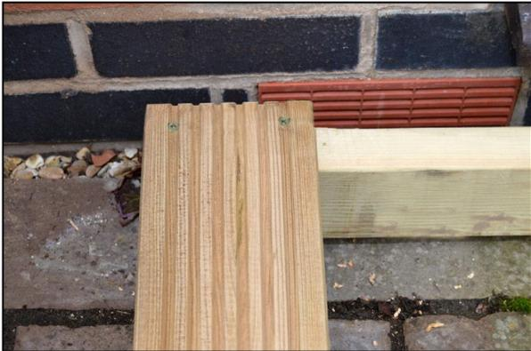
Align the rear facing end of the same section in place, again aligning its outer edge with that of the frame section before securing in place with 2 x shorter green screws.
