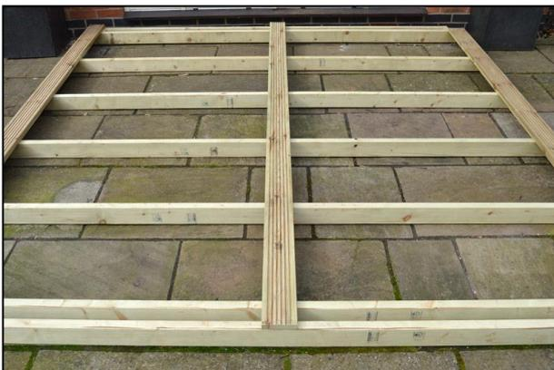
Take one of the decking sections and place it centrally across the joists as shown.
