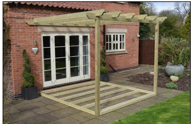
Add the remaining rafters, using the markings on the runner and wall plate to align them before securing in place with 2 x 120mm coach screws as per the outer rafters.
