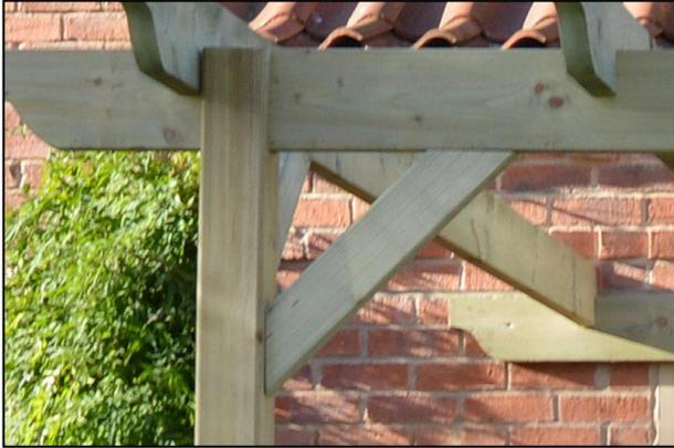
Position the short braces so that each end is flush a) with the inner face of the post and b) with the underside of the runner and centrally aligned before securing in place with a shorter screw at both ends.
