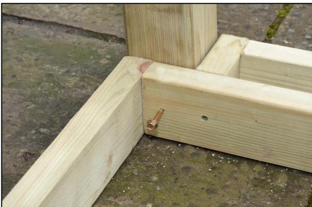
...before securing it into place with a 70mm coach screw through the pre-drilled hole in the frame front assembly. Attach the second post in the same manner.
