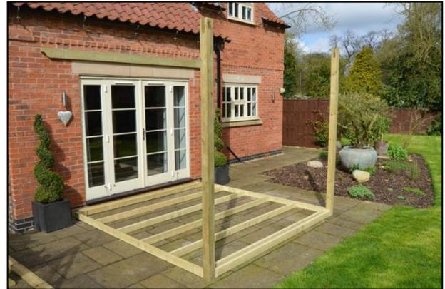
Get an assistant to hold a post upright in the pocket at the front corner of the base frame. Make sure that the notch in the top of the post is correctly oriented so that it is parallel to the wall plate...
