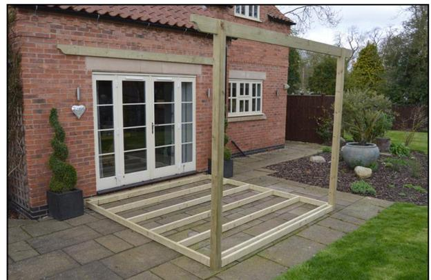
With the help of an assistant, slot the remaining runner into the top of the posts, using the markings on the runner to correctly align it centrally across the structure.
