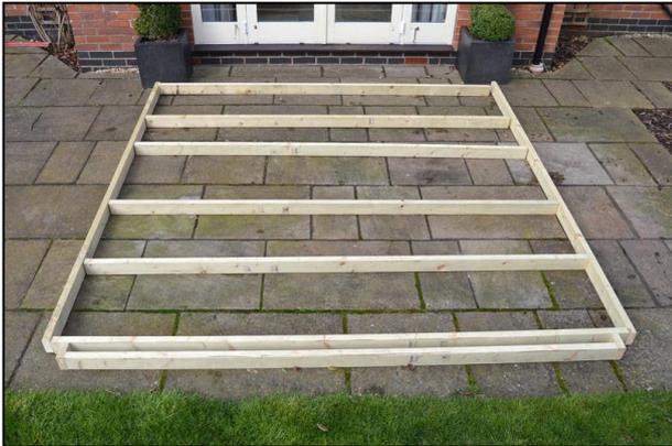
Lay out the base components adjacent to the wall where your wall plate is mounted. The base front assembly should be furthest from the wall and oriented as shown. The 5 joists should be roughly aligned to the markings on the 2 base frame sides.
