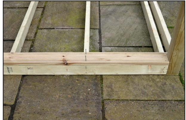
Work your way down the edge section, keeping it flush with the frame and using the joists as a guide, affix in place with 2 x shorter screws at every joist. Repeat Steps 20 -22 for the other decking edge section.
