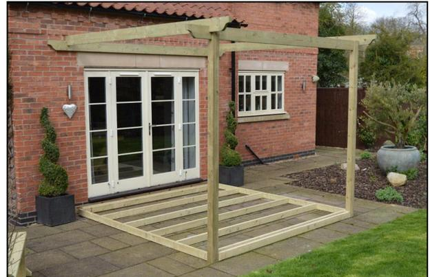
Now sit the outer rafters in place so that the inner face is butted against the post at the front and the rear is resting on the wall plate, aligned with the corresponding markings.
