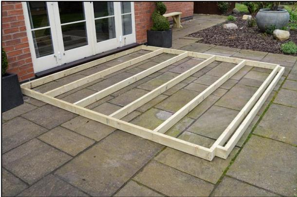
With the base assembly complete, slide it into place against the wall. To ensure it is central on the wall plate, mark the centre of the wall plate and the base frame and drop a plumb line from the wall plate - adjust the base position until the line and centre mark coincide.
