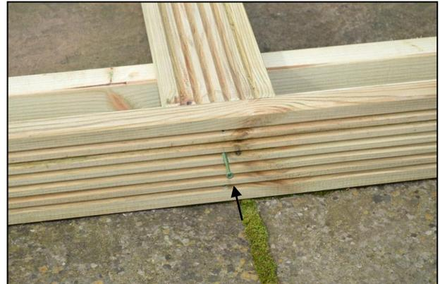
Using the decking section that you placed centrally earlier as a height guide, fix the centre of the front cladding in place, flush with the top surface of the decking using a shorter green screw.
