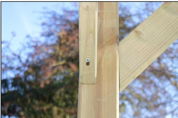
... and the bottom 45° face with the post, making it flush with the outer edge of the post before screwing the top and bottom into place with 3 x longer screws - 2 at the top and 1 at the bottom (do not over tighten).
