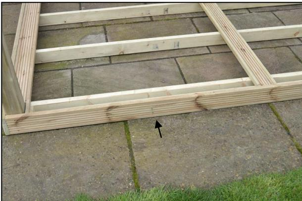
Add intermediate screws through the front cladding into the frame.
