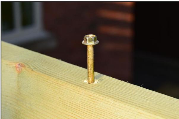
Fix the first rafter into place with a 120mm coach screw down through the top face into the wall plate at the wall end and into the runner at the other.
