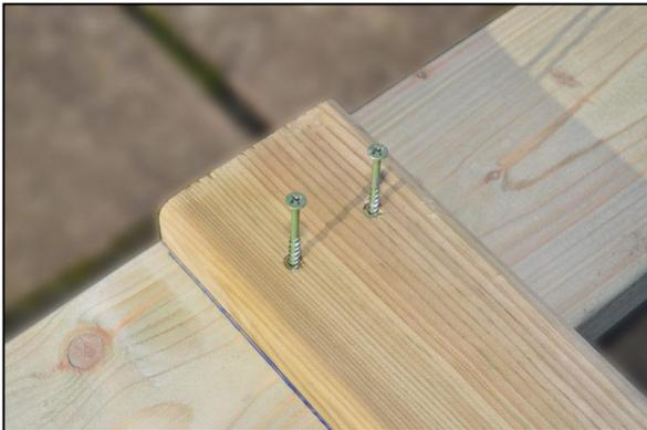
Fix the runner in place with 2 x longer green screws through both post tops as shown.
