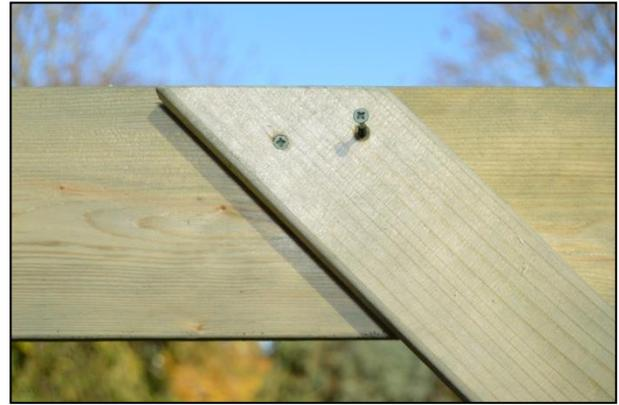
Now attach the longer braces by aligning the top 45° face with the inner top edge of the rafter...
