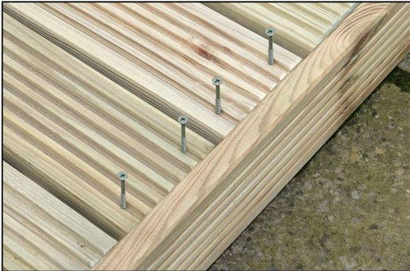
Fix the decking sections into place, using the frame joists as a guide for the screw spacing, with two screws at the edges and at each joist intersection.
