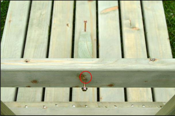
Ensure that the brace is lined up centrally on the table and attach it to the A-frame with a 60mm coach screw.
