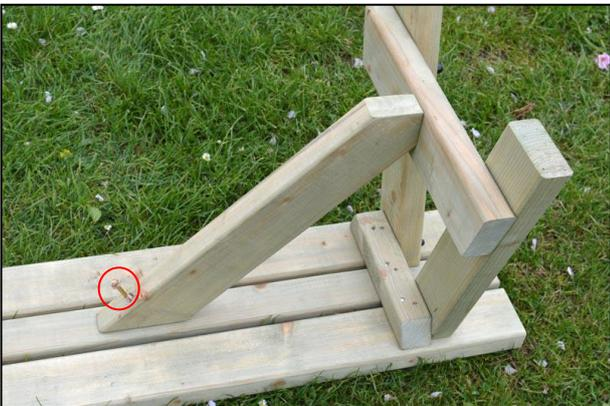
For a 5 to 8ft set, place a brace aligned centrally on the seat as shown and affix to the bench with a 60mm coach screw into the seat...
