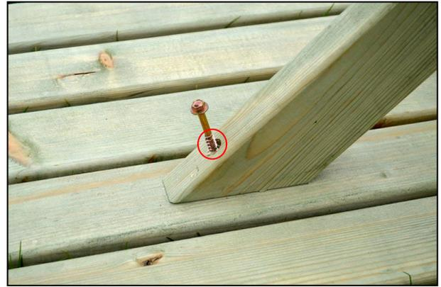
Make sure that the brace is still aligned centrally on the table and affix the other end to the table top with a 60mm coach screw as shown. Repeat steps 3 -6 to finish the table assembly and proceed to step 7.
