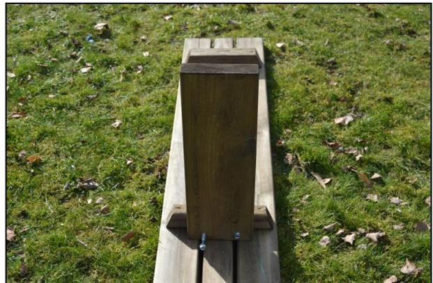
...and aligned centrally on the seat panel before fixing into place with 2 x 60mm coach screws as shown.
