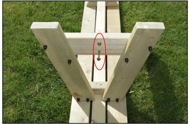
...before securing into place using 2 60mm coach screws at either end as shown.
