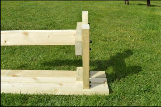
For a 3 or 4ft set, take one of the bench braces and align it between the two A-frames...
