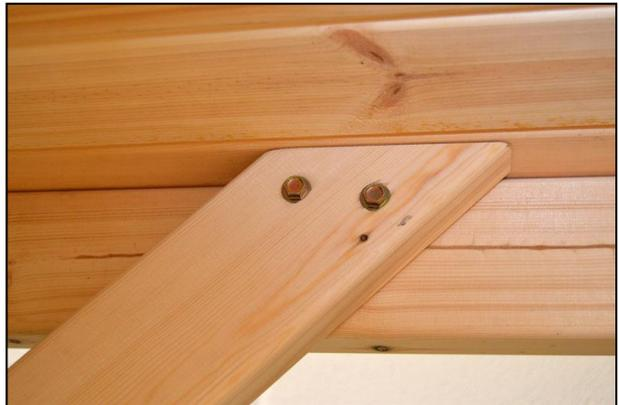
...and the other end is snug against the underside of the bench top. Secure the top of the brace using 2 x 60mm coach screws...
