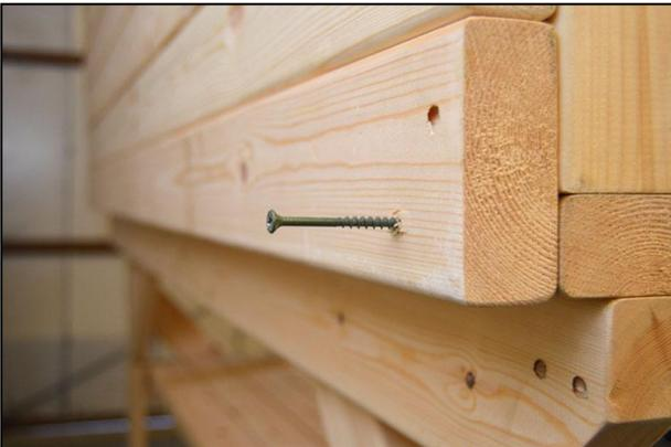
...and secure into place using 4 x 75mm screws. (45mm screws for MDF version)
