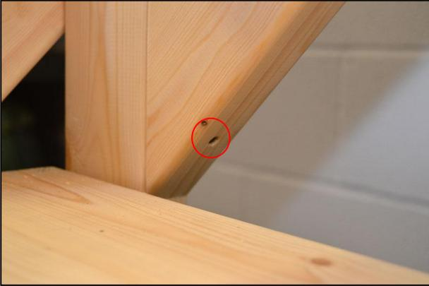
...and the lower end using a 75mm screw as shown here.
