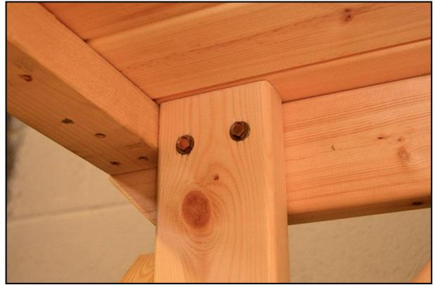
...and working from underneath the top ensure the top of each leg is located as shown, butted against the inner edges of the top before fixing each leg into place with 2 x 60mm coach screws.
